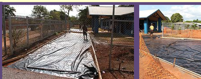
Preparation for concreting (Injinoo Day Care Centre).
