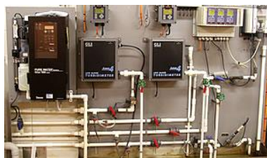
Above: The pH balance and chlorine levels are monitored here.
