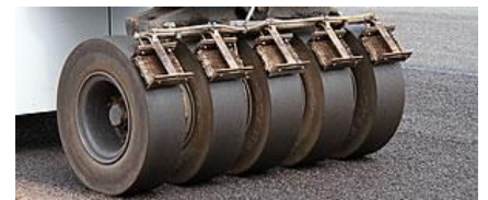
Rollers press the aggregate into the hot tar.
