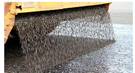
The aggregate is spread on top of the tar (the tip-truck is reversing).
