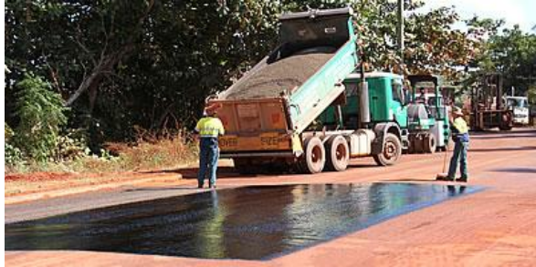
Fixing smaller sections in Seisia prior to the re-seal works.
