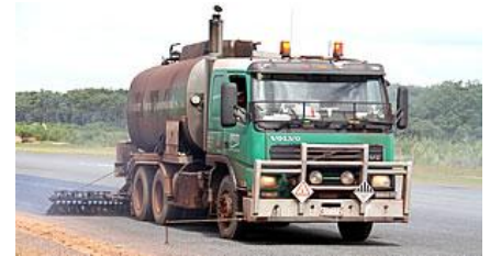
Hot tar is sprayed onto the surface.
