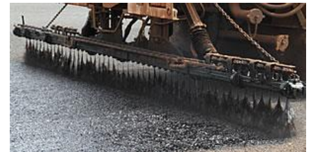
Hot tar is sprayed onto the surface.
