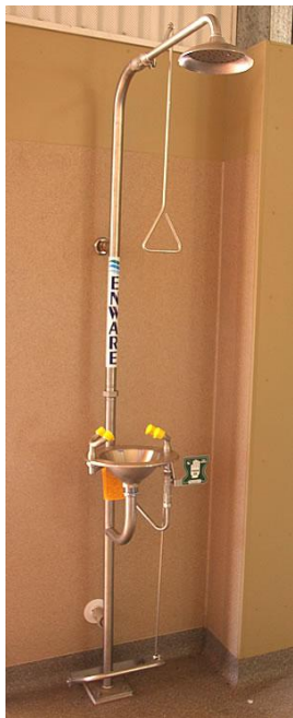
Eye wash and decontamination station.
