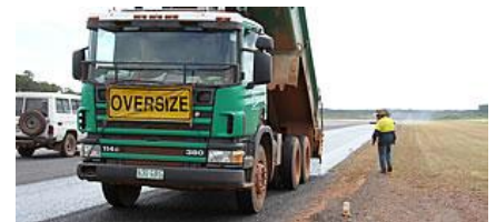
The aggregate is spread on top of the tar (the tip-truck is reversing).
