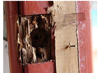
Crowbar marks, timber missing, latch was found on floor.
