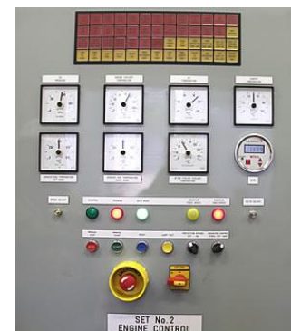
Left: These are the analogue read-outs from one generator set.
