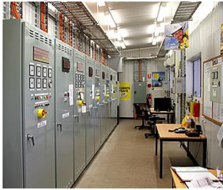
The control room. The cabinets on the left house the analogue displays of each of the generator sets.
