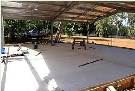
...the rear wall being sheathed. The sidewalls will be fly screened.
