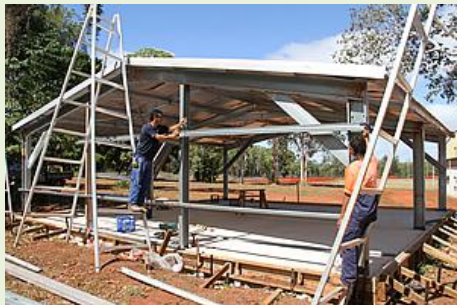
...the rear wall being sheathed. The sidewalls will be fly screened.
