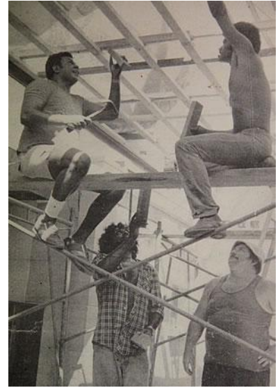
The description with this image reads: Six months earlier, these boys hardly knew what a hammer and nail looked like. Under the expert guidance of TAFE instructor Bill Hourigan (lower right), Edward Dau, Bagai Seriat (both on the plank) and Joseph Asai fix ceiling battens in the major upgrading of the Cowal Creek canteen. Local labour is employed on a big program of building works in the Northern Peninsula Area.
