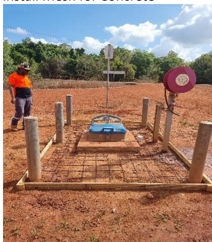
Install mesh for concrete
