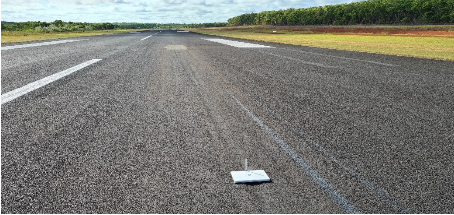
Figure 21 existing impact ruts on runway
