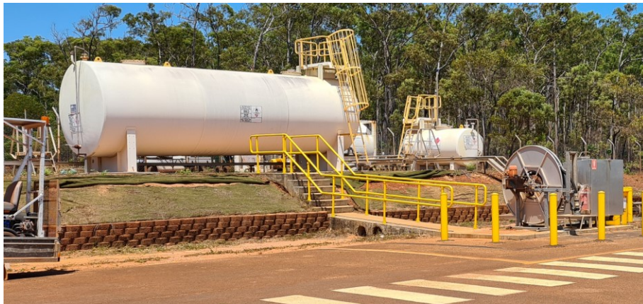
Figure 61 Jet A1 and Avgas refuelling facility
