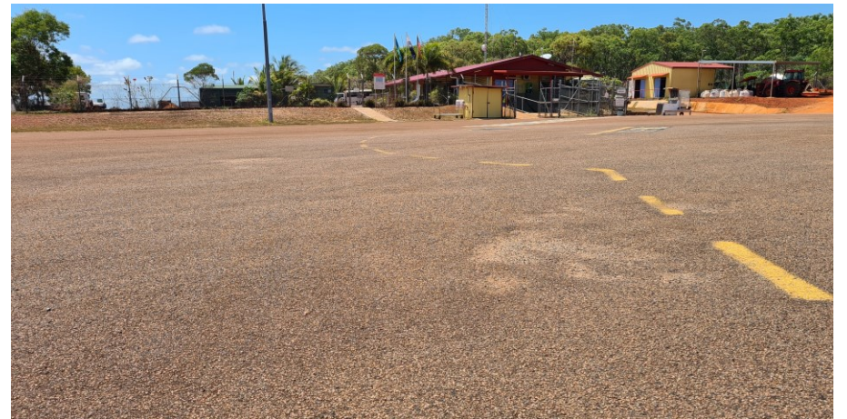
Figure 24 Main parking apron pavement deformation
